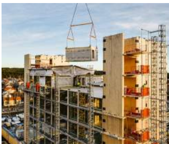
Sara Kulturhus in Sweden features over 10.000 m3 of timber including CLT elevator shafts. Design: White Arkitekter Picture: Martinsons/Jonas Westlin
