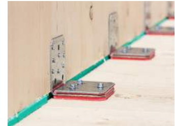
Elastomers added under CLT slabs and metal connectors.
