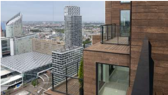
Thermally modified compressed bamboo as applied at the Grotius residential towers in The Hague. Design: MVRDV Picture: MOSO International
