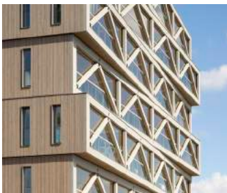
Patch 22, a hybrid timber building features a glulam post beam structure with a demountable prefab concrete flooring system. Design: FRANTZEN et al. Picture: Luuk Kramer
